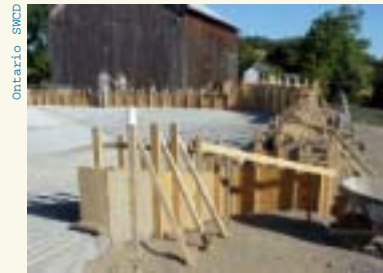
Construction of a barnyard runoff management system.
