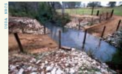
Completed stream crossing.
