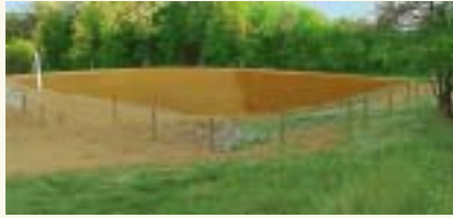
Construction of an agricultural waste system.
